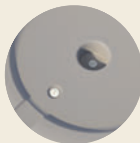
OVERFLOW HOLE AND RESERVOIR DRAIN HOLE
