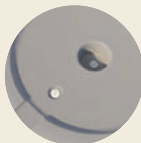
OVERFLOW HOLE AND RESERVOIR DRAIN HOLE
